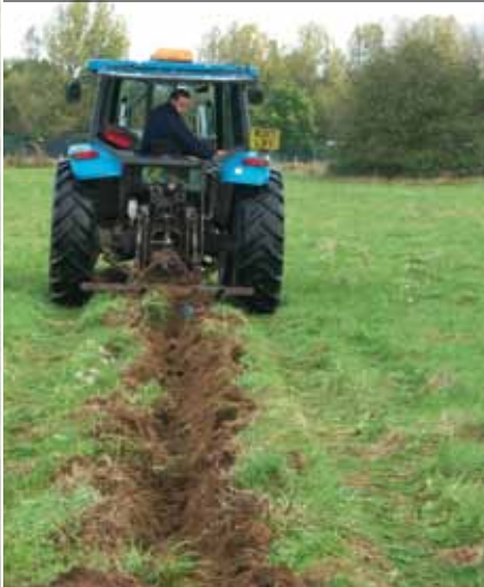
Creating foot drains using a tractor. © River Nene Regional Park (RNRP)
